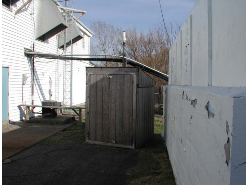
Figure 13: Lidar and Security Enclosure at the WBZ Data Validation Test Site
